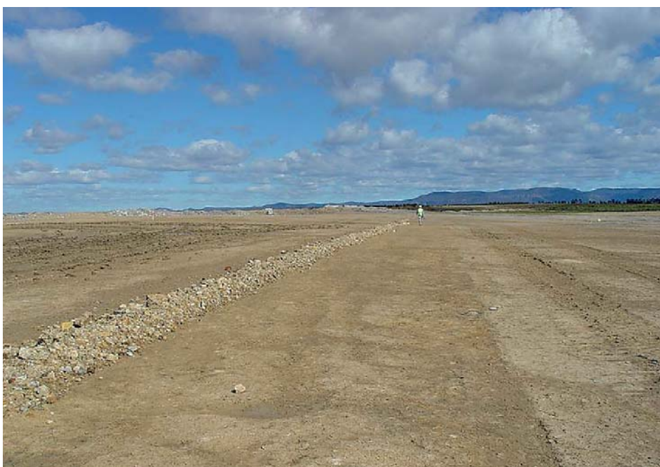
Plate 2. Reshaped overburden ready for revegetation
