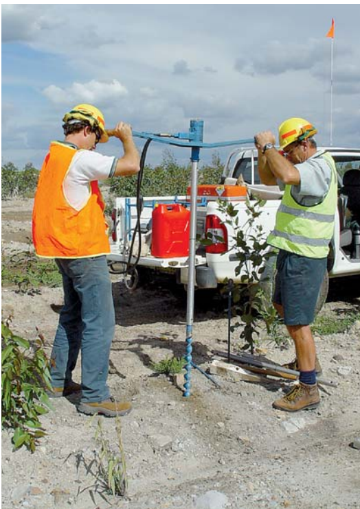
Plate 16. Installing Neutron Probe Access Tubes
